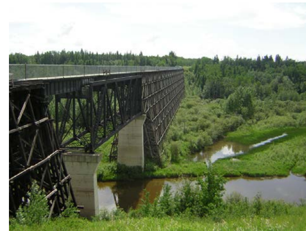
Beaver River Trestle, Alberta's Iron Horse Trail
